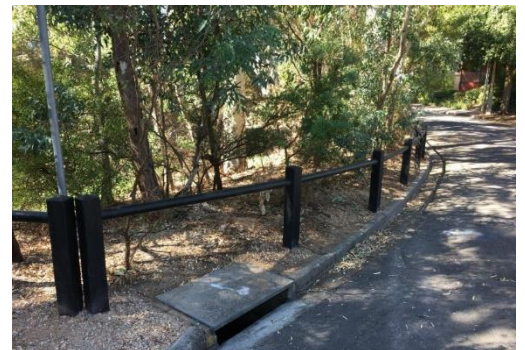
Recycled plastic bollards have been used extensively by Australian councils for over 30 years in rural & bush applications.
